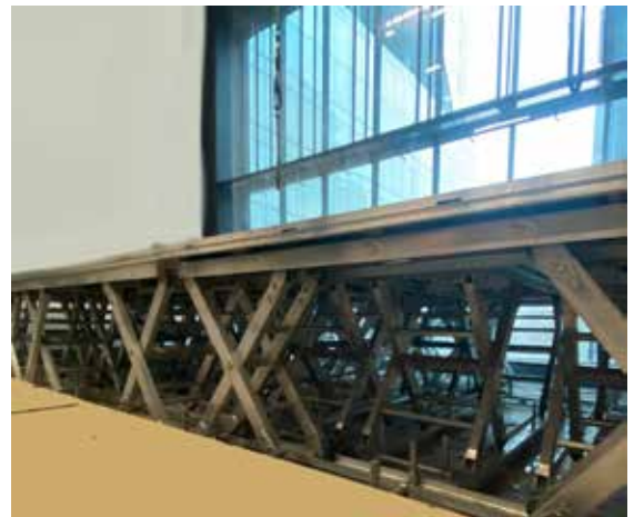
SHOWLIFT DURING INSTALLATION AT MASSEY HALL
